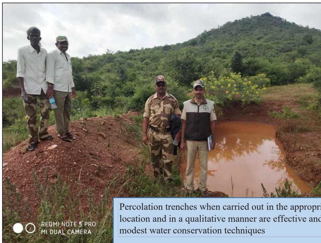
Photo 5: Hyrada Block 2 Plantation, Hadagali range, Ballari division & circle Percolation pit filled with water having stabilised bund indicating appropriate location
